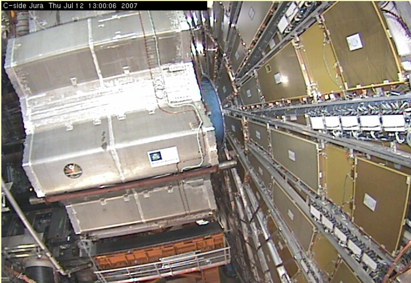
Installation of the second (last) endcap toroid: 12. July 07
